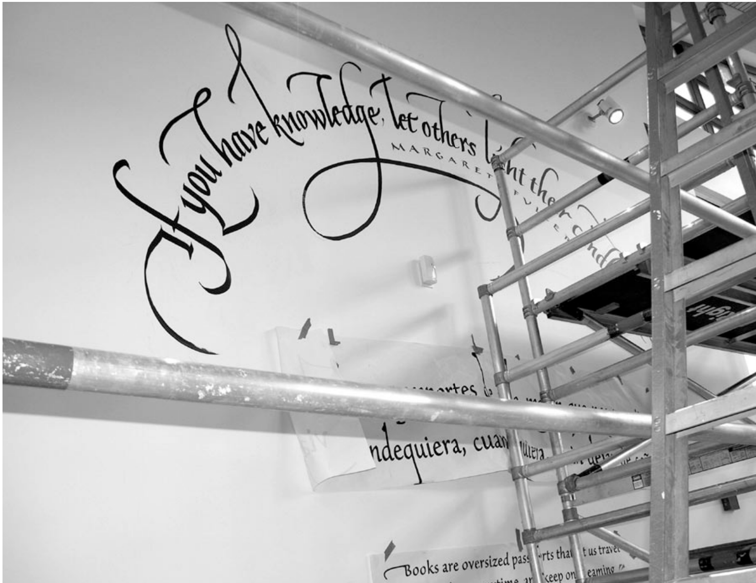
Two tiers of scaffolding at the Belmont Library.
